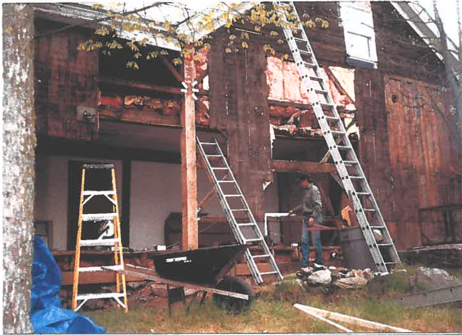
Lloyd Remodeling Barn
